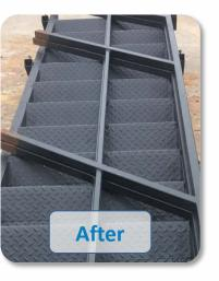
**ShieldTec Epox-600** is a unique water based one pack epoxy gloss coating that can be applied direct to metal and over rust making it ideal for refurbishment for metal applications. ShieldTec Epox-600 provides superior adhesion with an extremely tough and hardwearing decorative finish. This fast drying finish provides good anti-corrosive properties and is easy to apply by spray, brush or roller.
